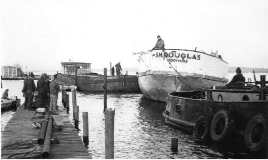
SM Douglas being placed in line with the Irving Barge.
