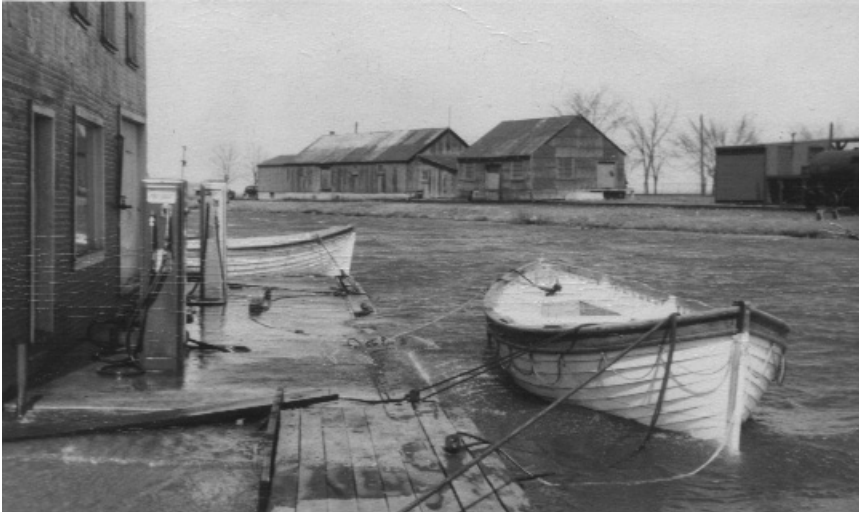
1950's View of the original clubhouse buildings on Blockhouse Island in Tunnel Bay from the gas docks at St. Lawrence Marina looking east. Note the high water, probably in the early spring. The land in front of the buildings was leased from the CPR and the buildings purchased for $1500 in the mid 1950s. It was an early beginning for the eager sailors of Brockville and area.
