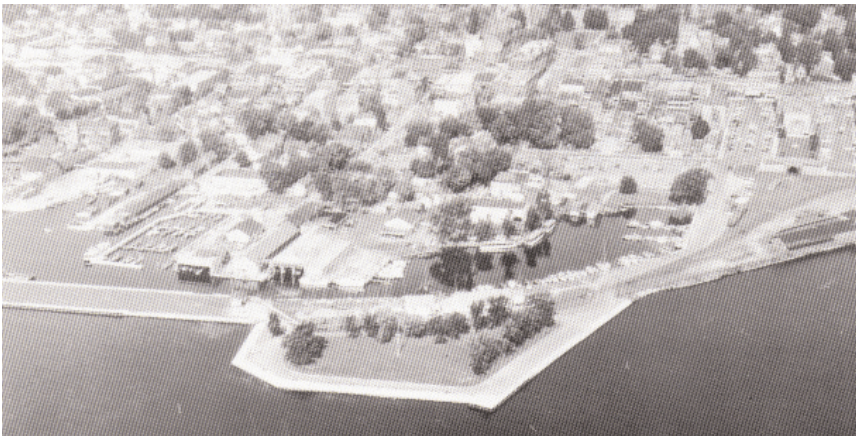
Aerial view of Brockville Yacht Club on Blockhouse Island, 1961.
