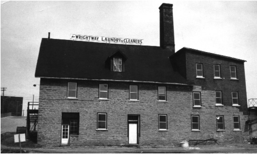
Wrightway Laundry before renovations begin.
