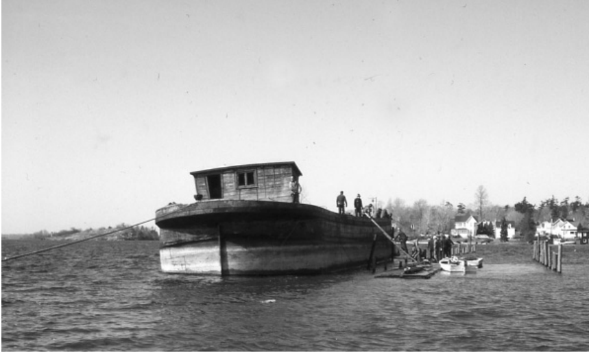
Irving Barge put in place as a breakwater.
